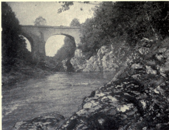
High Bridge and River Span.
